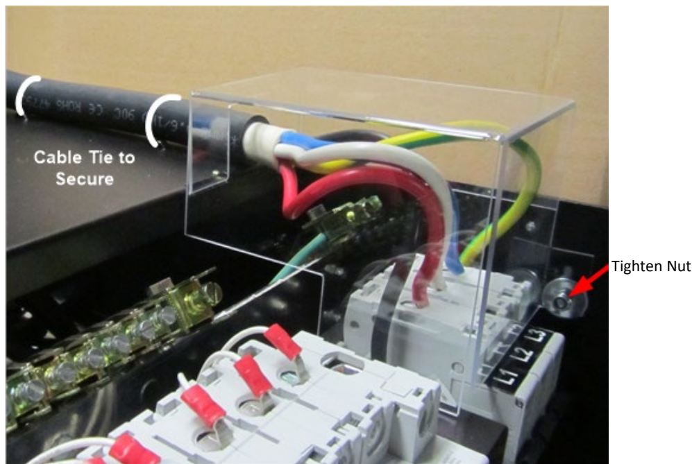
Figure 9: Lock the AC Terminal Cover
